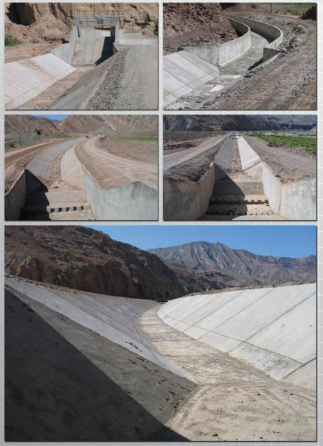
Including :Construction of the canal (ave. length :6774 meter ) , Angled drops (30 no. ) , Concrete culverts (10 no.) ,Overpass bridges in form of aquaduct (ave . Length : 50 meter) , Containing Wall (ave. length : 3750 meter), Concrete Siphone (ave . Length : 250 meter ), Covered concrete box (ave. length 400 meter )and intake structures( 4 no.)
