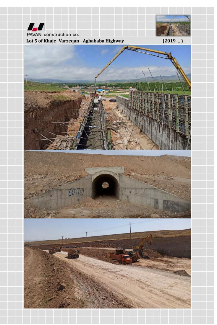
The Fifth Section of Khajeh-Varzaghan-Aghababa's highway (from kilometer 50+200 to 61+550) is located in East Azerbaijan province. This project is approximately 11,350 meters length, with the final width of 15 meters. It includes 11 meters of asphalt roads and two gravel shoulders, each with the width of 2 meters. Subgrade construction, base, asphalt, and technical structures are as follows:
